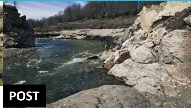
Demolition of the Retuerta Dam on the Aravalle River (Spain)
